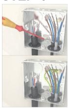
Depending on the mat supplied the cold tail from the cable has an earth which is a braided wire or solid earth cable. If it is necessary to shorten the cold tail, at the thermostat, then the earth braid must be 'unpicked with a small screw driver or similar tool.
